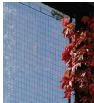
This glass noise barrier was made visible by using wire networks. 3
