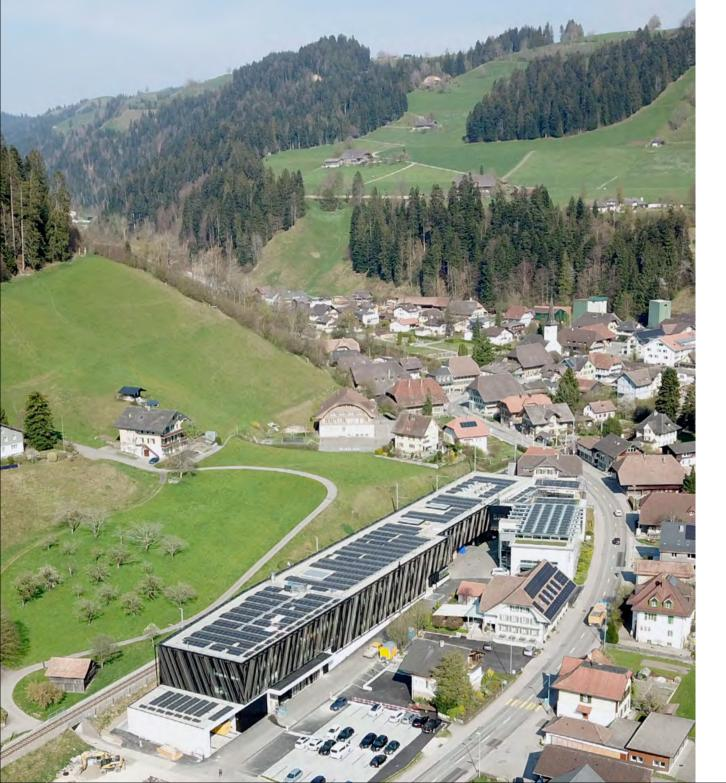
All roof surfaces in Trubschachen are fully equipped with modern photovoltaic systems. This gives us a total solar power output of 350 000 kWh per year.
